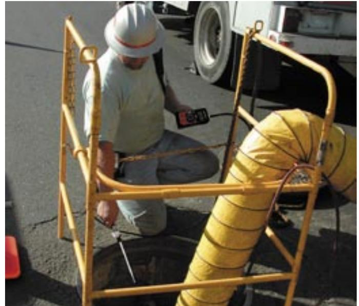
Once the lid is removed, the sample probe can then be lowered into the confined space starting at the top and sampling all levels until the probe reaches the bottom.
